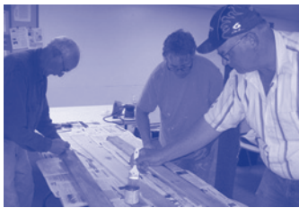
Preparing the chair railing
