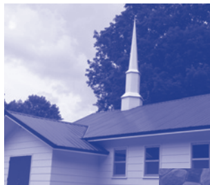
New roof on Limestone Baptist Church
